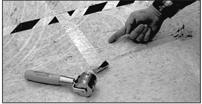
Figure 2. Grounding Strips Installation
