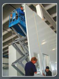
Panel Replacement: The non progressive post design provides the ability to swap or replace individual panels without disturbing the adjacent panels.
